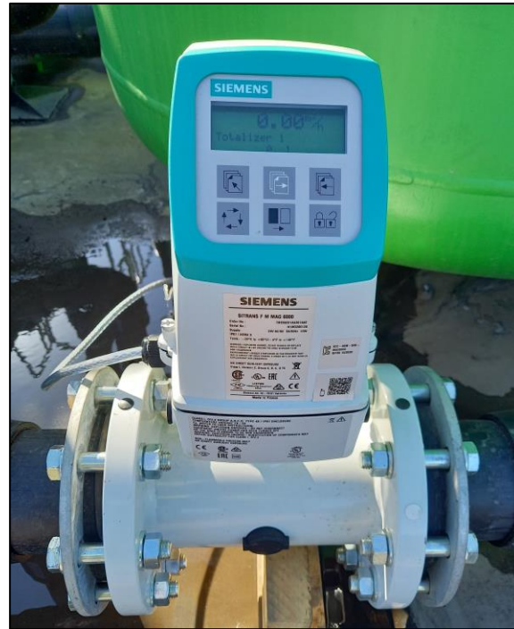
Figure 14. Electromagnetic flowmeter
