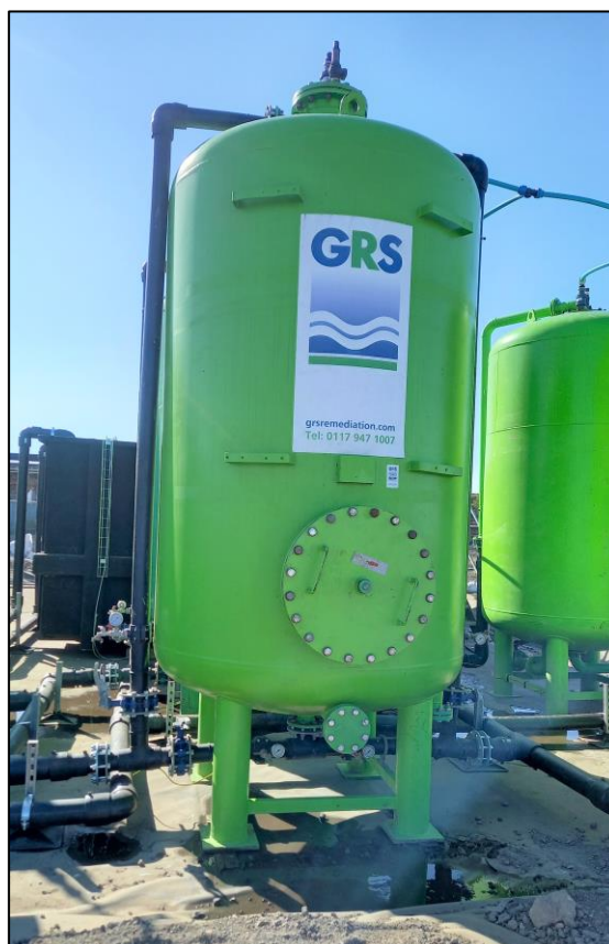
Figure 10. BI50 carbon vessel (GAC)
